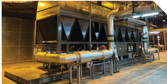
Large-scale chiller replacement project
