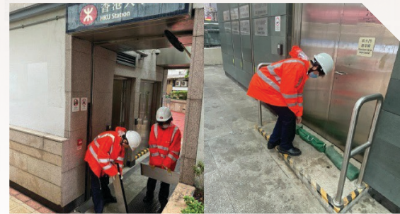
(Left) Operating colleagues installed flood boards at stations; (Right) Operating colleagues placed sandbags outside stations to prevent rainwater from entering
