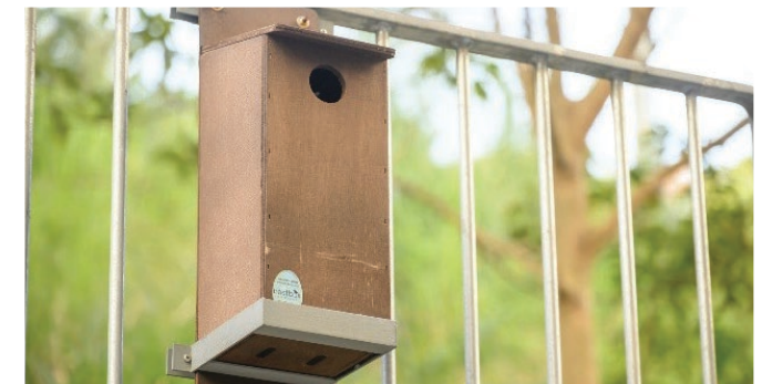
Bird nest box installed in Hin Keng Station
