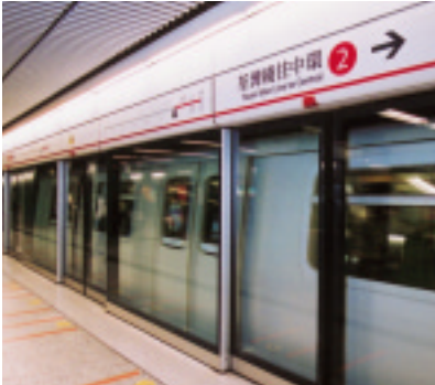
February New platform screen door at Tsim Sha Tsui Station
