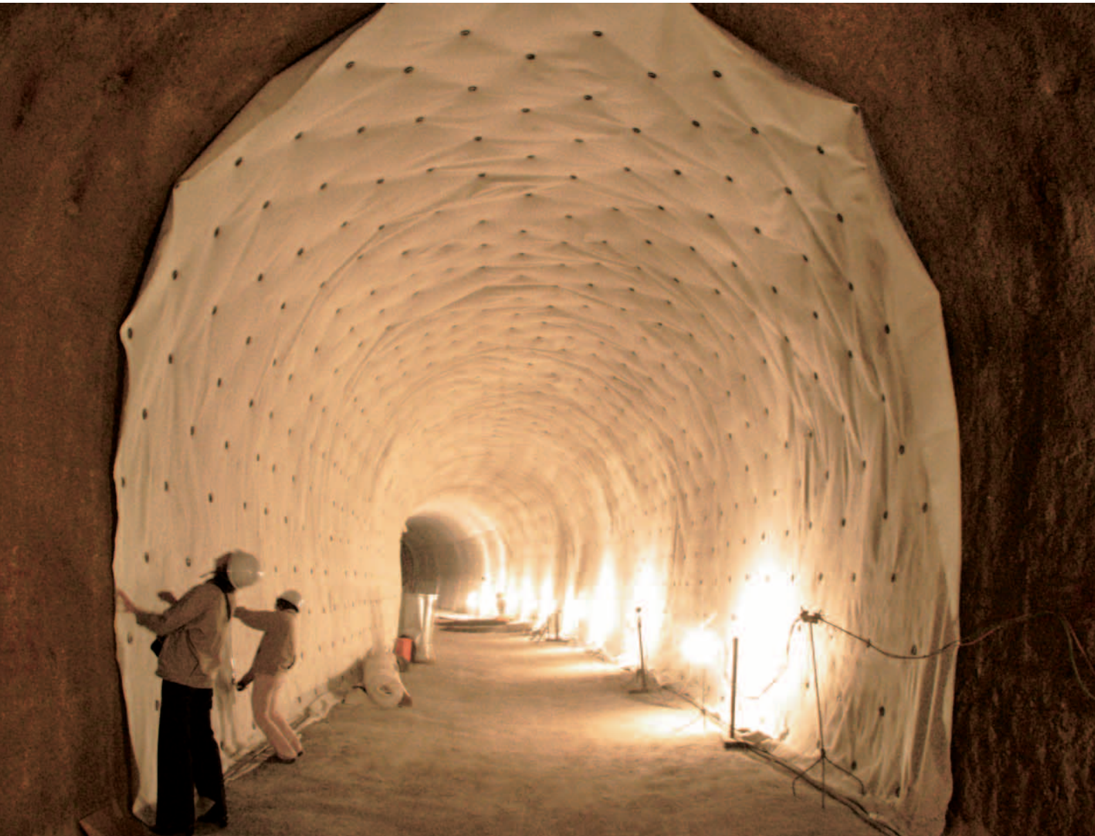
14 stations have been handed over to the B JL4 PPP company to start E&M installation
