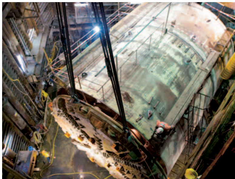
Construction works on the Kowloon Southern Link
