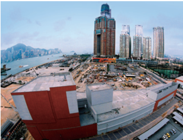
Kowloon Southern Link will connect East Rail Line to West Rail Line in West Kowloon.
