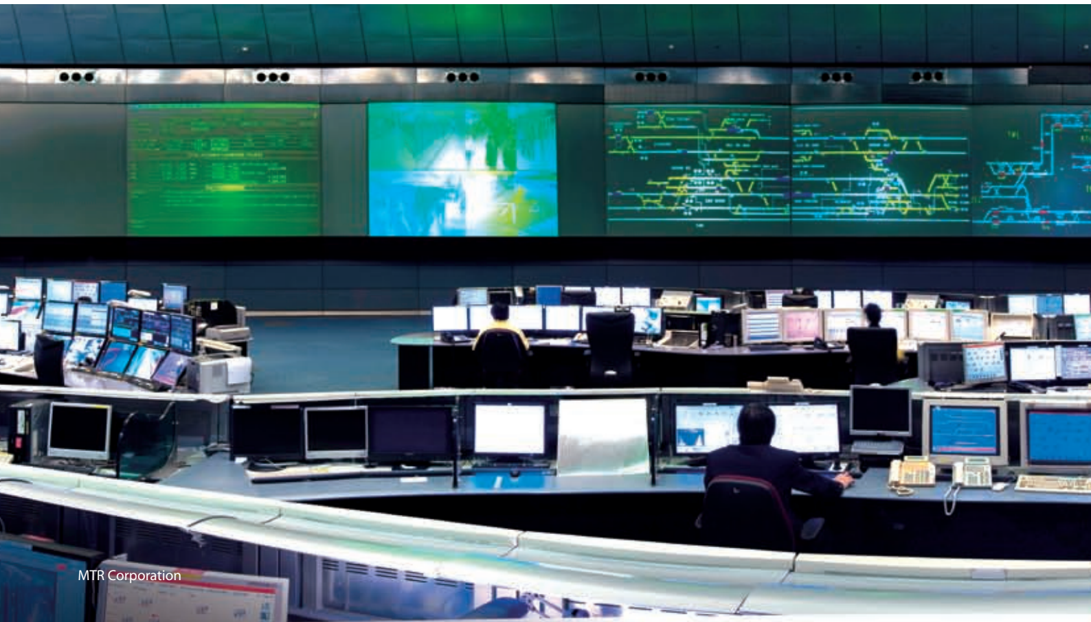
Our Operations Control Centre in Tsing Yi monitors train operations.
