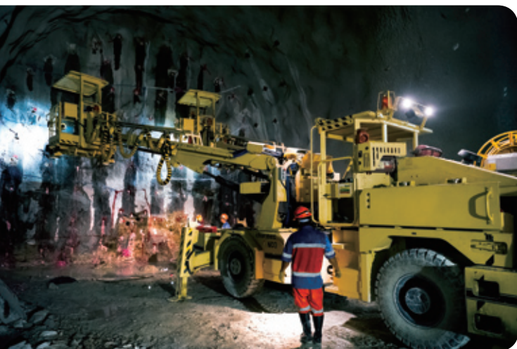
Massive tunnel drilling jumbos are working underground in the "drill and blast" sections for the Express Rail Link
