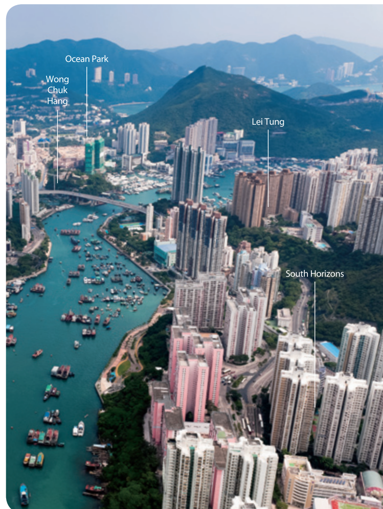
The South Island Line (East) will provide railway services to the Southern District of Hong Kong Island
