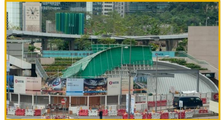
Construction Site of SCL at Admiralty Station
