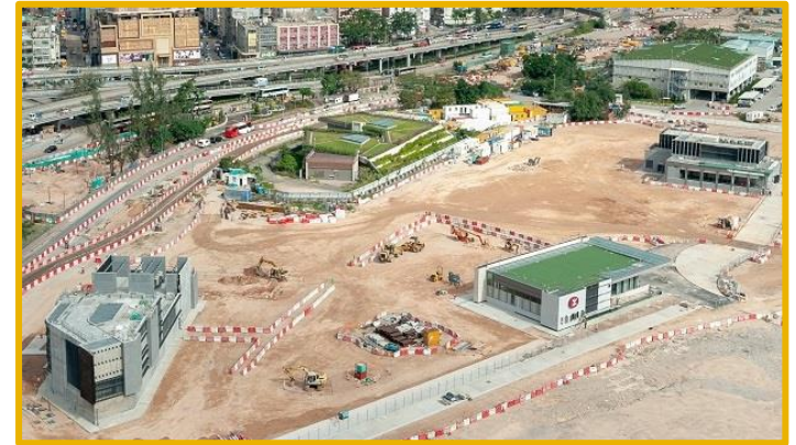
Sung Wong Toi station
