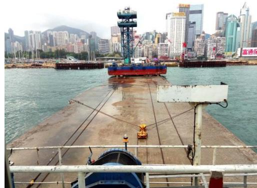
The Shatin to Central Link (SCL) will provide a fourth cross harbour rail tunnel for Hong Kong. With the successful installation of the last Immersed Tube Tunnel (IMT) pre-cast unit for the cross-harbour rail tunnel in the Victoria Harbour on 12 April (Thursday), the immersion works of all 11 IMT pre-cast units have been completed. This is a significant step forward in the construction of the SCL project.
