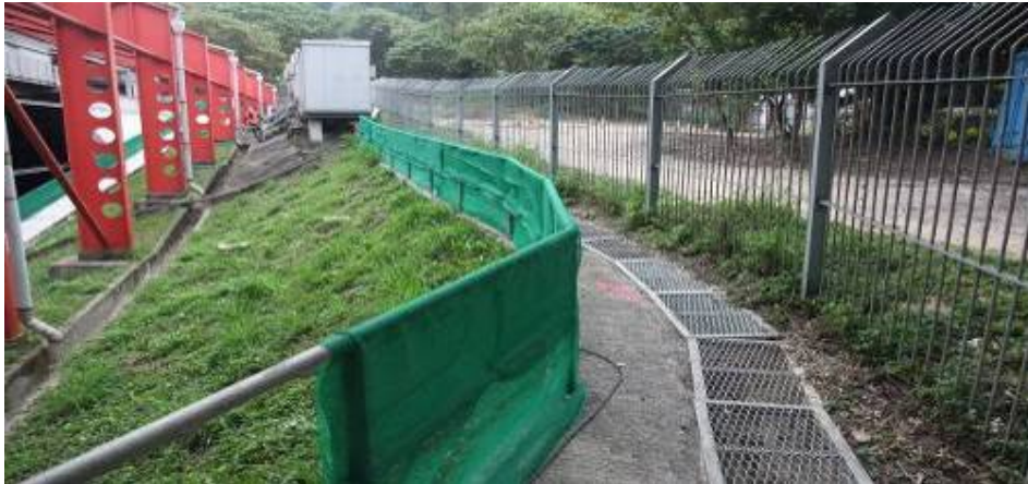
改善前 Before Improvement
