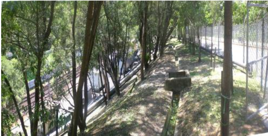
改善前 Before Improvement
