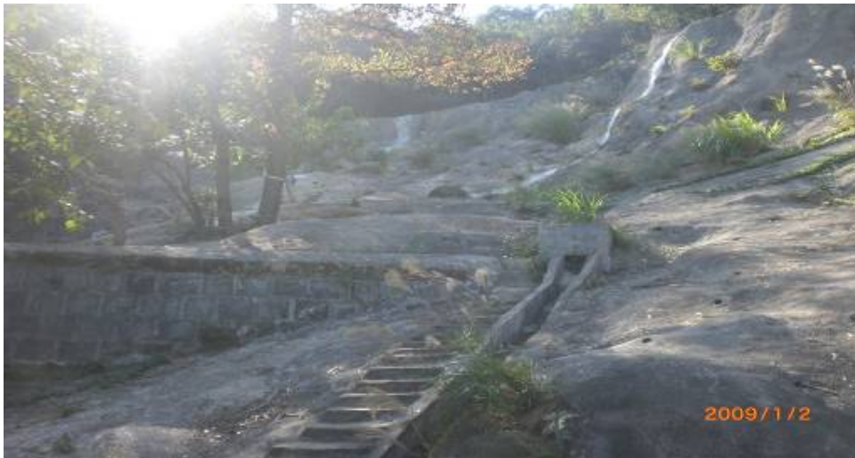
改善前 Before Improvement
