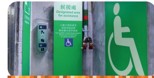
The design of the Refuge Area is in compliance with proven international standards and meets the safety requirements of government departments. Passengers in need can contact staff from the designated area with the Helpline.
