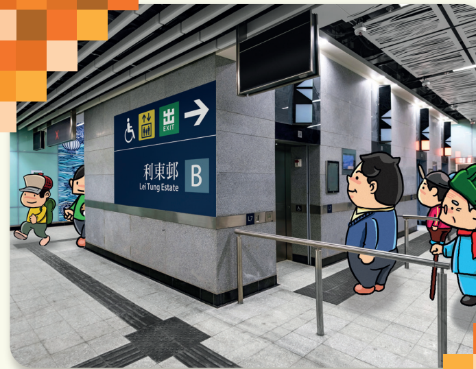
Each lift is designed with doors on two sides to separate in and outflow of passengers, ensuring a smooth passenger flow.
