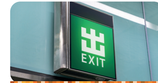
When the station system detects an Emergency, flashing exit and directional signs, as well as public announcements will divert passengers away from the incident location and show the way to the nearest exit.
