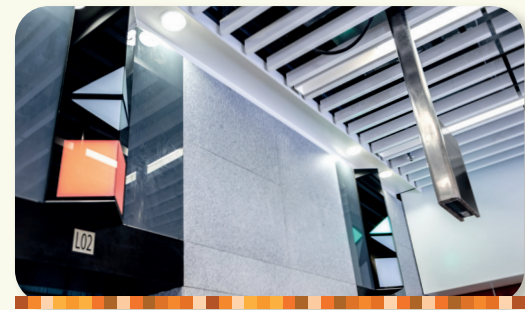
Lights on the lift indicate its direction. Green when the lift is going up, red when it is going down.
