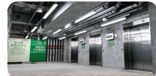
The Refuge Area is constructed with fire-resistant materials which will stop the spread of fire and smoke into the Area. Passengers can leave the station using the lifts in the Refuge Area, or wait for assistance inside the Area. Emergency staircases to the Ground Level are also available.
