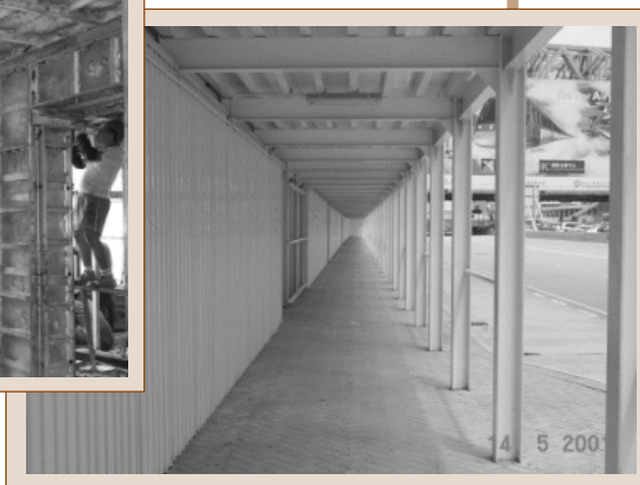
▲ Metal hoarding adopted in construction site
