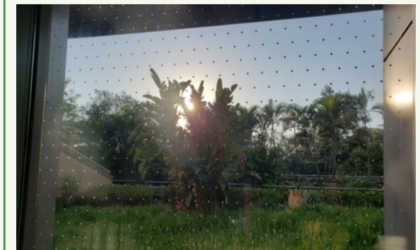
Installation of anti-bird collision window films on over 100 window facades in Mei Foo Station
