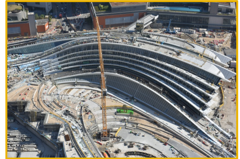
West Kowloon Station
