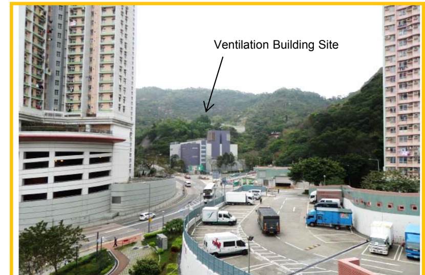
Yau Tong Ventilation Building Site
