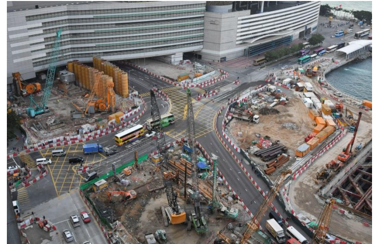
Exhibition Station Site
