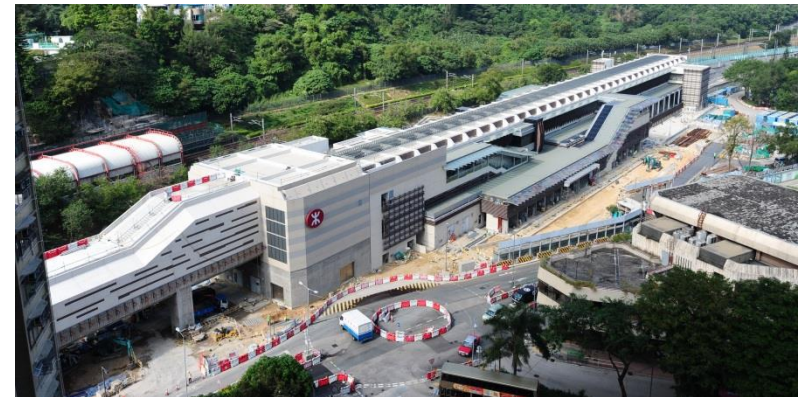
Hin Keng station
