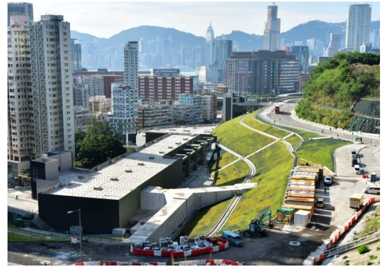
Ho Man Tin Station Site
