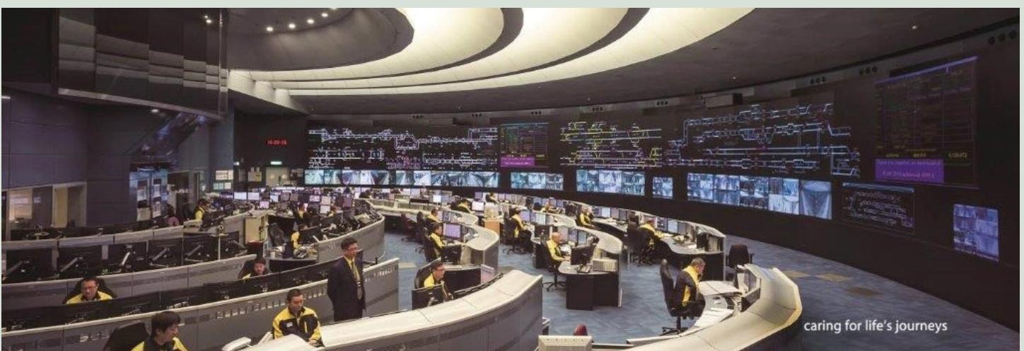
Our Operations Control Centre (“OCC”) controls the Hong Kong rail network from Tsing Yi
