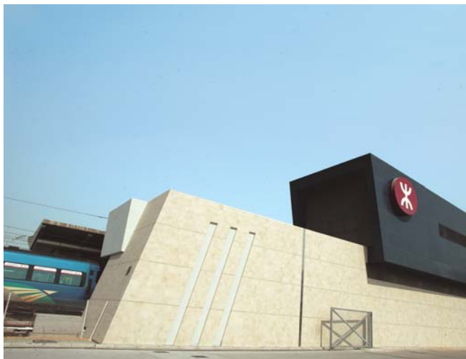
Integrated with AsiaWorld-Expo, the new AsiaWorld-Expo Station provides a convenient and direct access to the Hong Kong's newest and largest exhibition facility via the Airport Express Line
