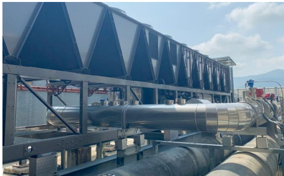
Chiller replacement at Kam Sheung Road Station
