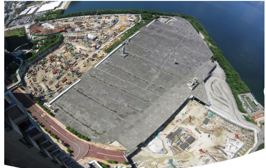
LOHAS Park Packages 4, 5, 6 & 7 under construction
