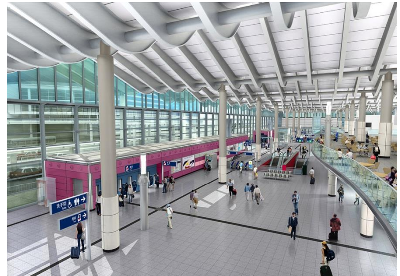
The new Hung Hom Station concourse after improvement works
