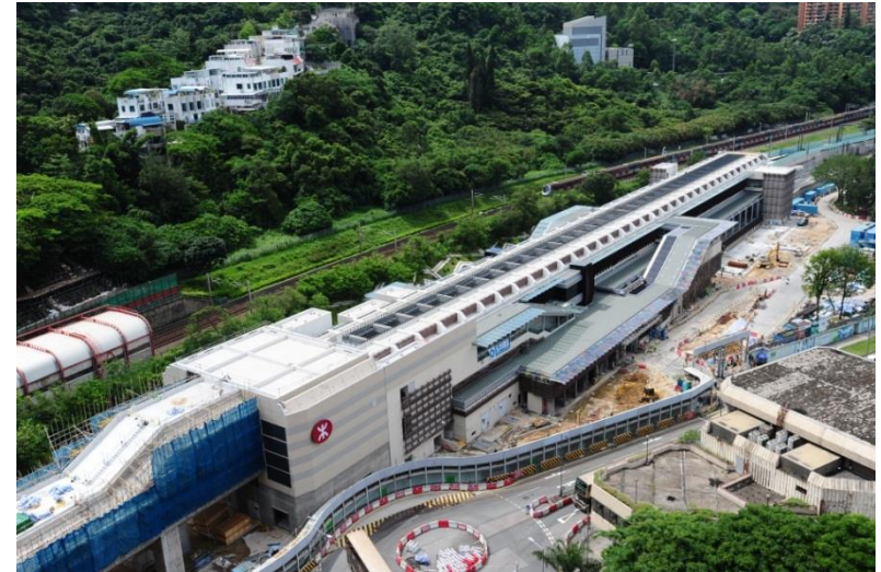
Hin Keng Station
