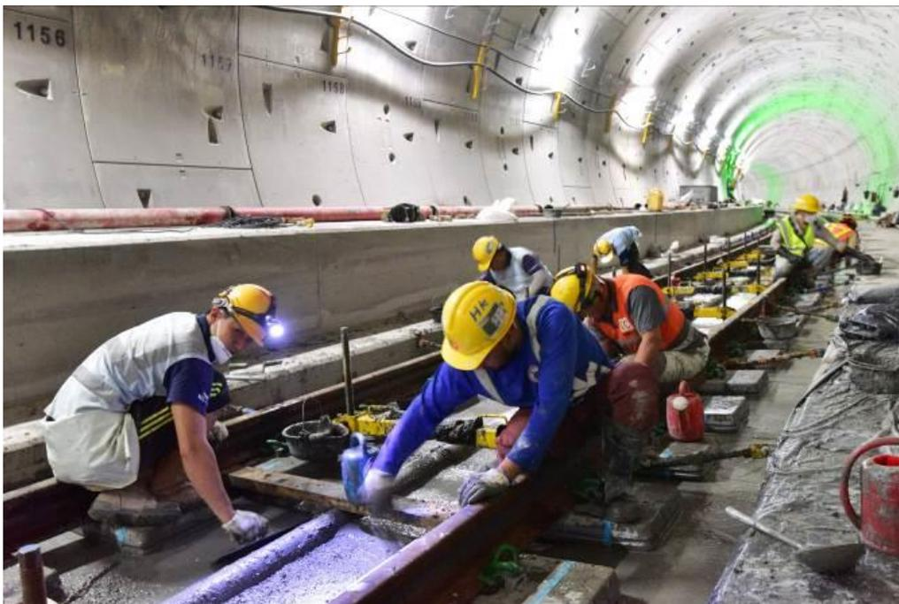
2. SCL on track: Works trains are now being deployed to facilitate track-related works at the East West Corridor of the SCL project.
