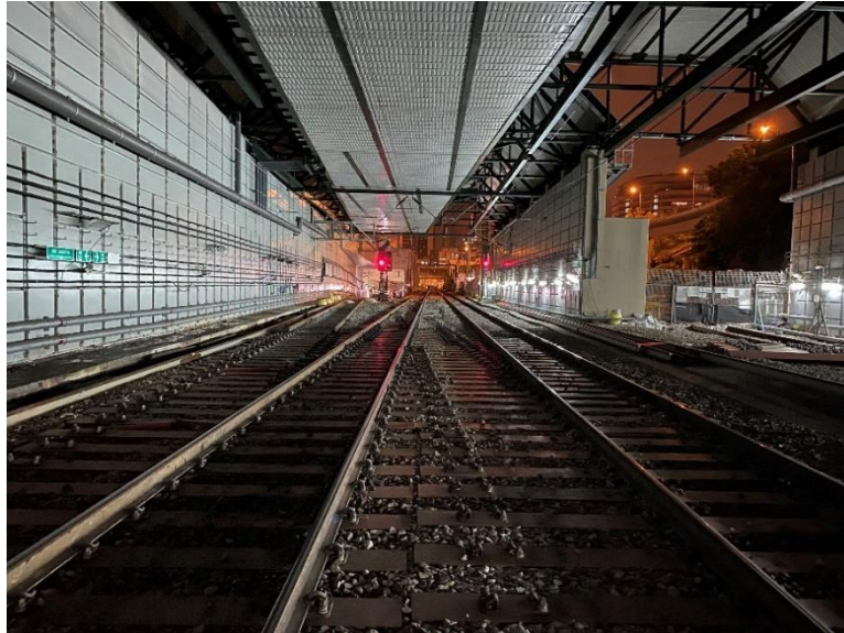
Before the works
