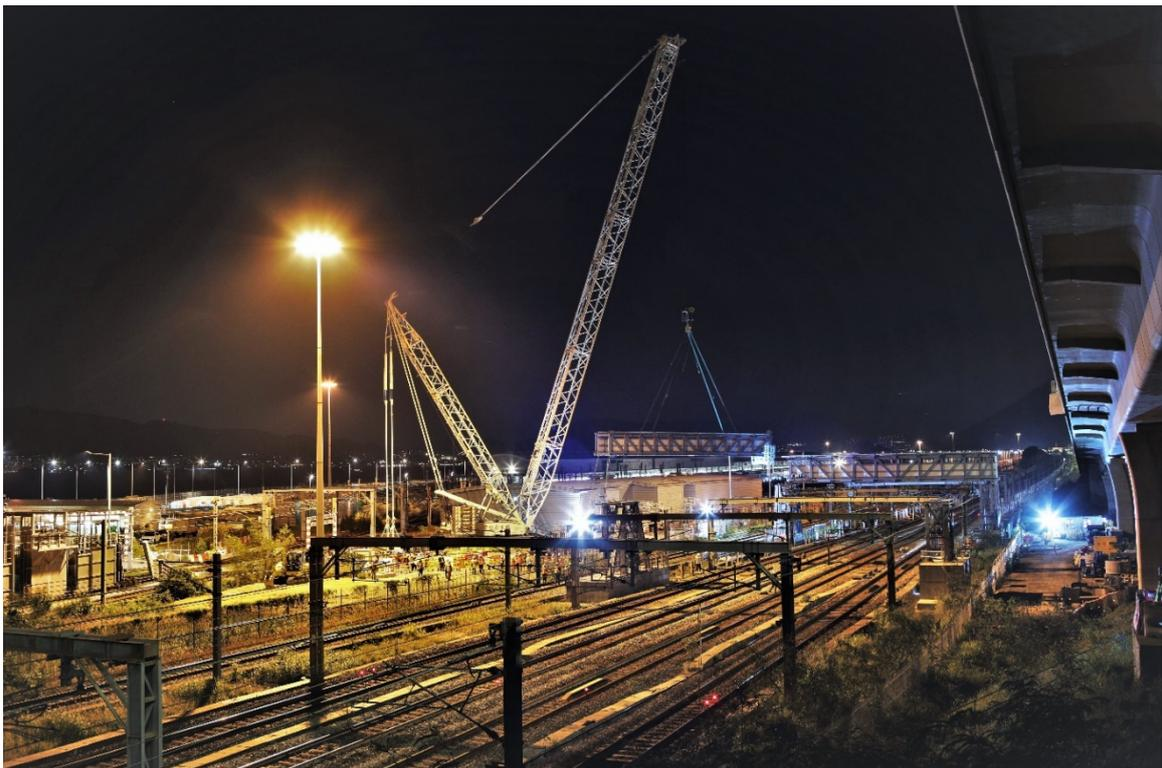
Through the two cable bridges, underground cables and utilities will be diverted and re-routed from near the Siu Ho Wan Depot to the other side of the Tung Chung Line and Airport Express Line tracks, allowing for subsequent development works atop the depot. The lifting and installation of the second cable bridge will be completed in January next year.
