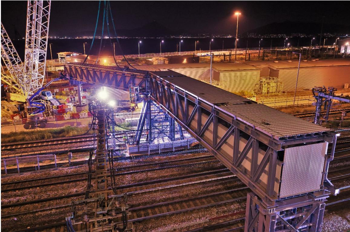
To ensure the safe and smooth completion of the heavy lifting and installation works within the very limited non-traffic hours, the engineering team prudently and carefully planned each step of the works, which was then thoroughly simulated and trialled with the contractor before the works were actually carried out.
