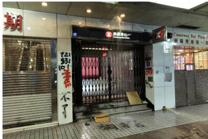
Entrance/Exit B of Causeway Bay Station
