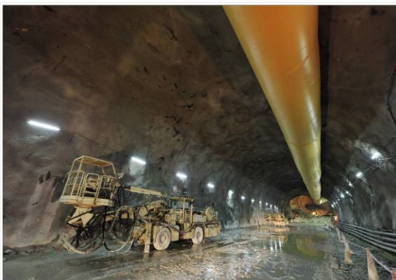
Typical drill and blast tunnel under construction
