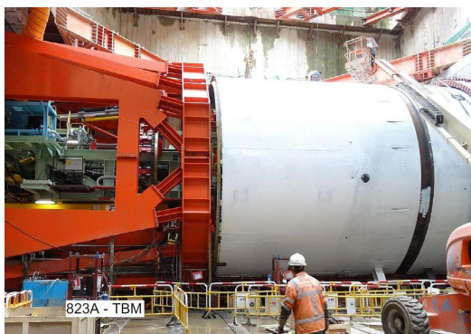
TBM at contract 823A
