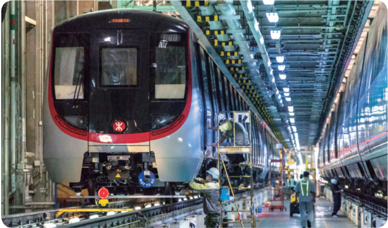
We spent over HK$6 billion on maintenance, renewals and service improvements for our railway assets in 2014
