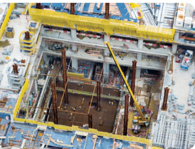
The overall excavation work of the West Kowloon Terminus was 88% complete by the end of 2014
