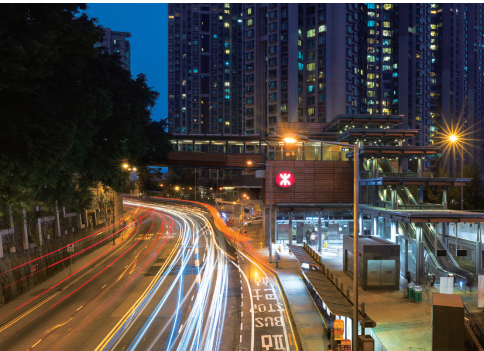
HKU Station on the Island Line extension opened for service in December 2014
