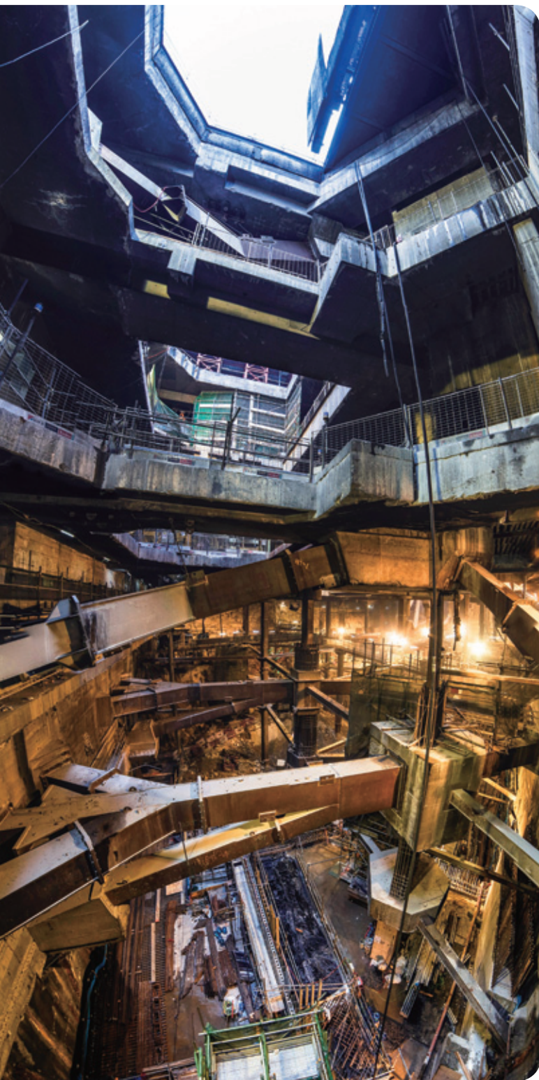
The technically complex works for the underpinning of the existing Island Line tunnel, in order to construct the extension of Admiralty Station, continue to be a major challenge
