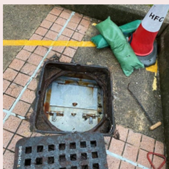
Installation of flap valves at the drainage pipe to avoid back flow of seawater.
