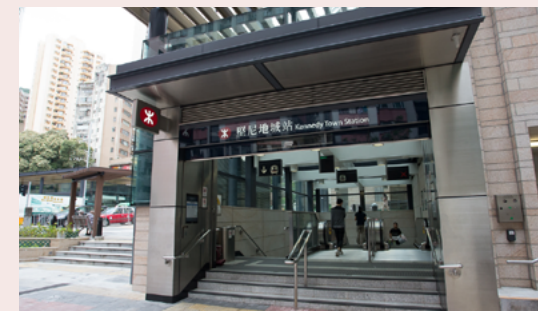
The entrances/exits of most MTR stations are by design at least 450mm above street level and equipped with 1.2m high flood boards.
