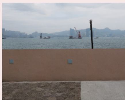
Planter walls at Heng Fa Chuen Playground to prevent the influx of overtopping wave water.
