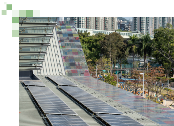
Solar panels installed at roof of Hin Keng Station.
