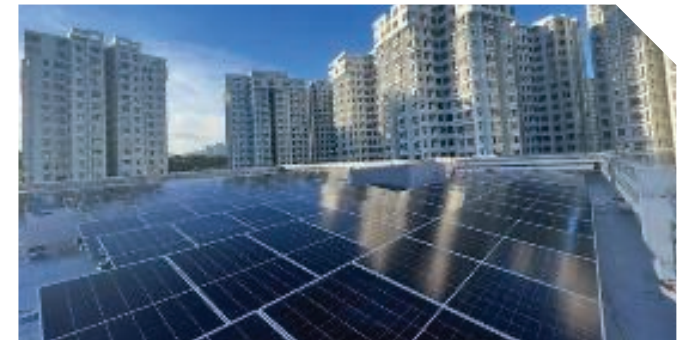
Installation of the solar panels at Paradise Mall
