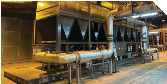
Large-scale chiller replacement project
