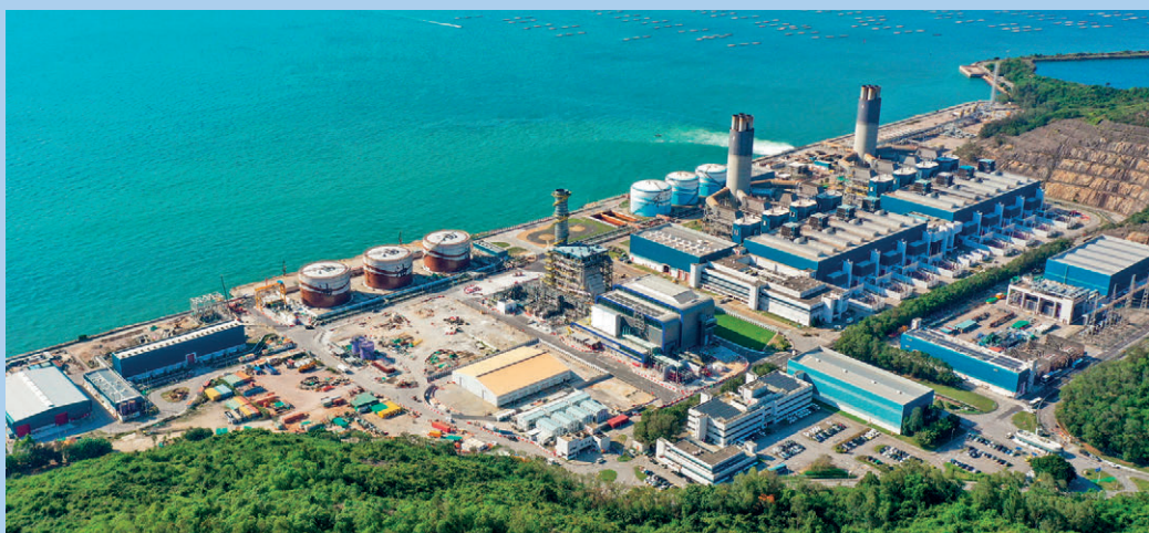
Black Point Power Station
