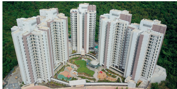
Fire Services Department Pak Shing Kok Married Quarters in Tseung Kwan O is the first batch of high-rise concrete MiC buildings in Hong Kong
