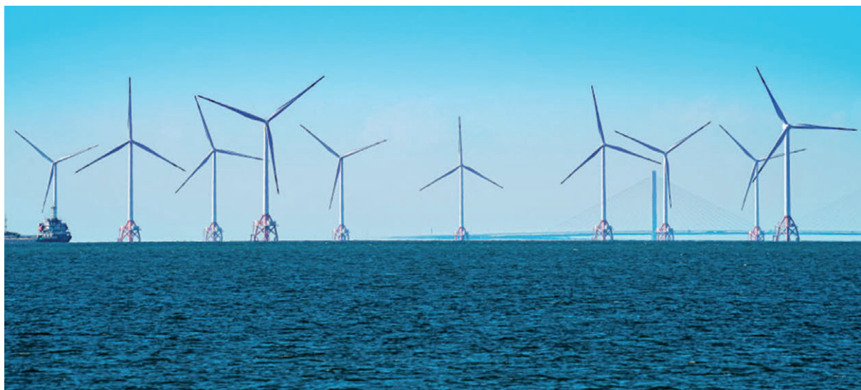
An offshore wind farm at the GBA
