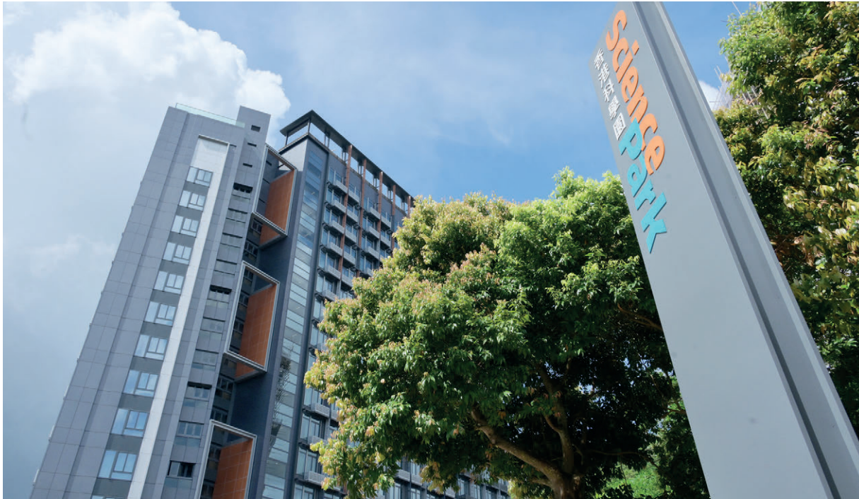
The InnoCell located in the Science Park is Hong Kong's first batch of high-rise building projects adopting MiC method
