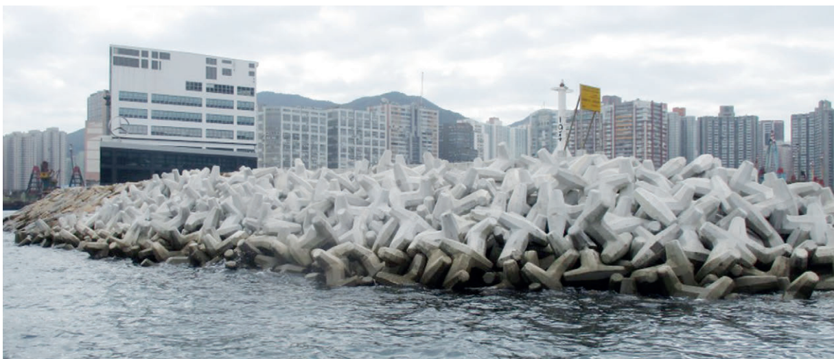
Chai Wan Breakwater
