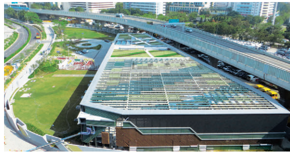
DCS at Kai Tak Development
