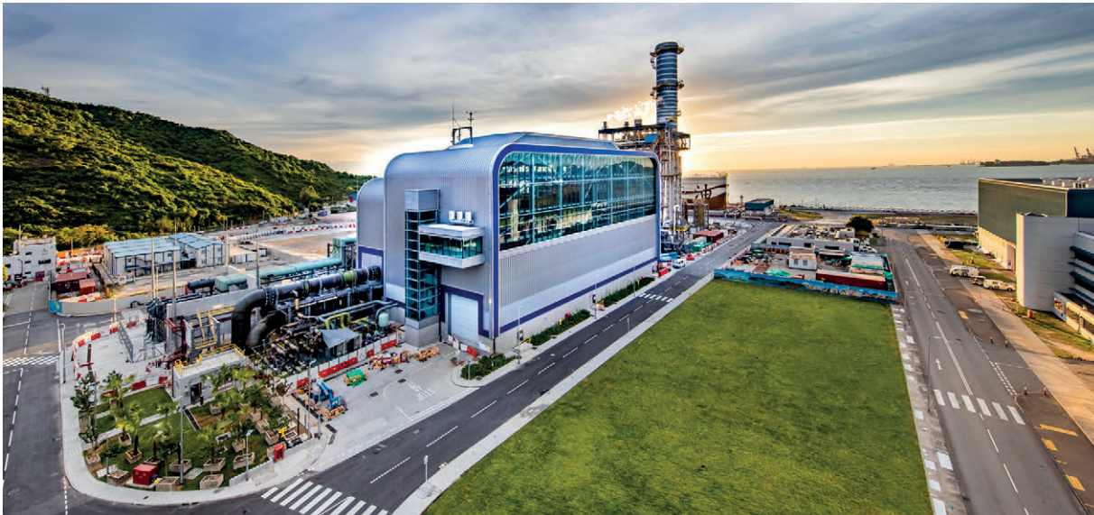
New gas-fired generation unit at Black Point Power Station
