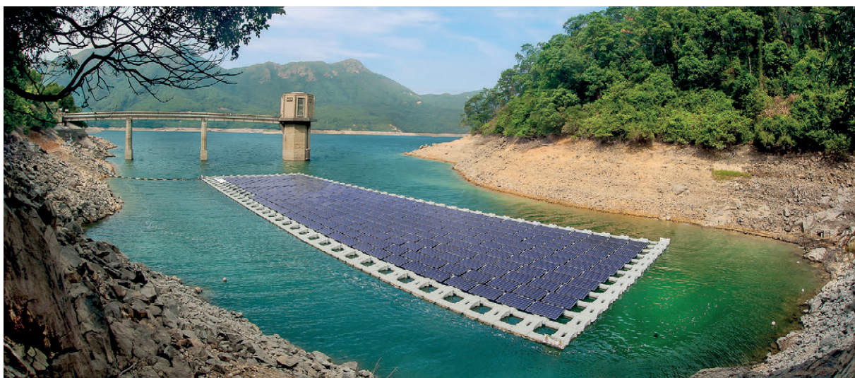
The floating solar energy generation system at Shek Pik Reservoir
